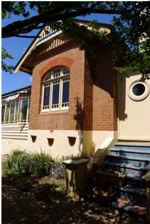
Figure 34: Original entry steps onto eastern verandah north of the central gabled bay. Some cracking is evident.
